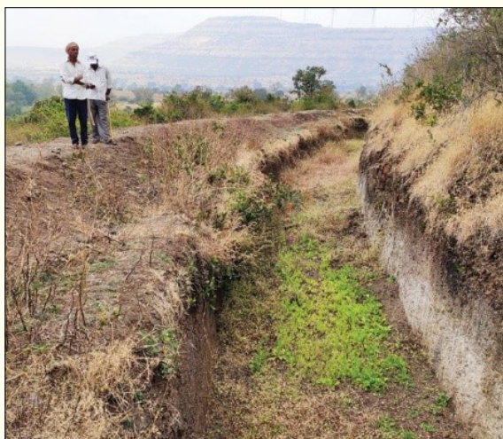
Observation of Water shed Area of Jaigaon during the exposure visit – (left) visit to deep CCT structure, and (right) farm ponds constructed to collect the rain water from the catchment area and used for irrigation purpose.
