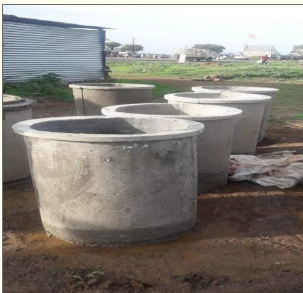
(left) Cement tanks used for soak pit under the Tank Model, (right) BJS field team marking out the pits for the construction of soak pits
