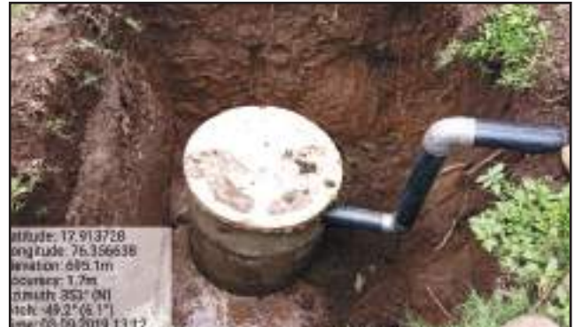
Two models of Soak-pits under construction in village
