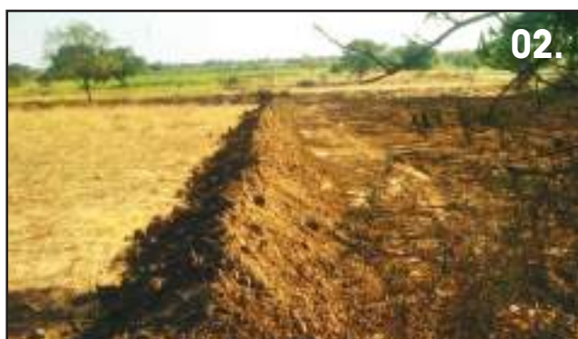
Pics 1, 2 and 3 - Different stages of Compartment Bunding
